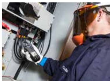
Analyze Power-related Issues
